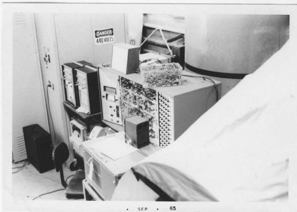
Hybrid computer, pilot control input recorder, gimbal power conditioner and controller.
