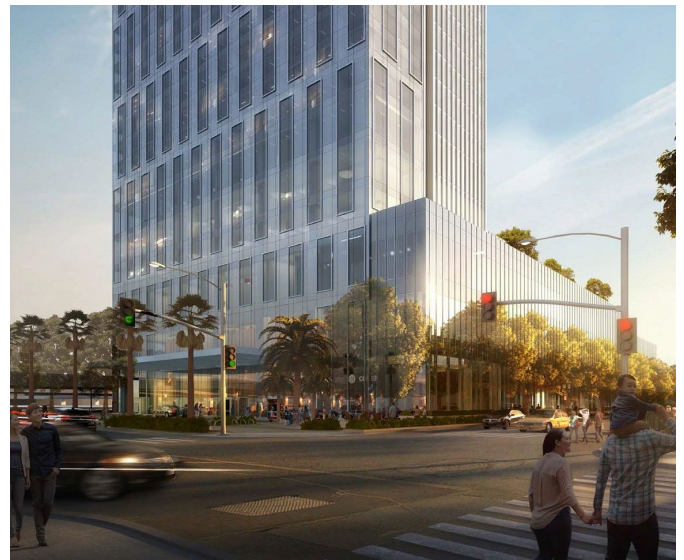
The Albany, LA Convention Center Hotel Los Angeles, CA
