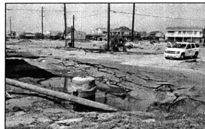
(b) Damaged Roads
