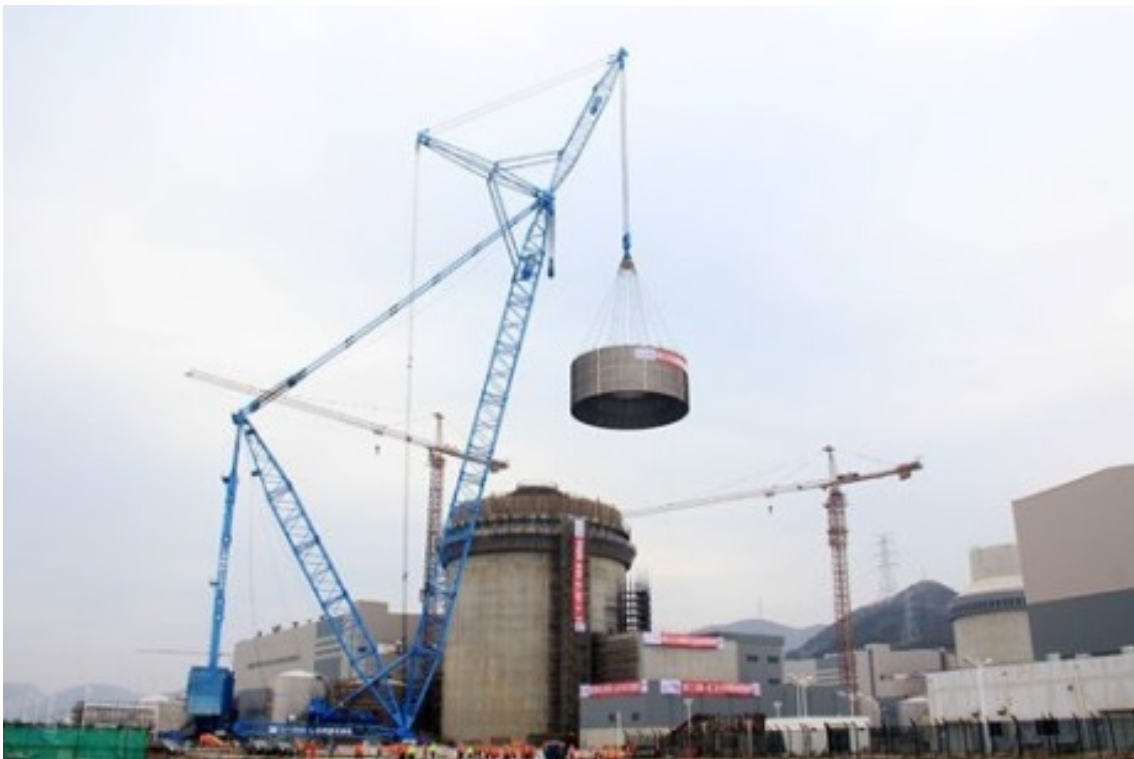
Figure 3.3: Installation of final module, containment water tank, at Sanmen 2 in China (01/2016) [2]
